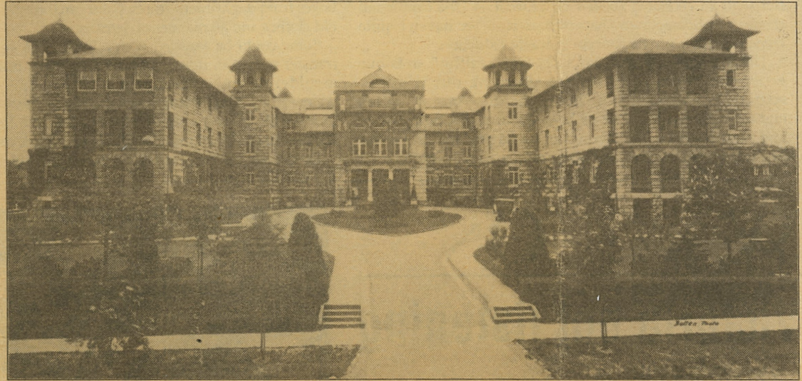
The Heather Pavilion in the 1920s, then the entire Vancouver General Hospital.
